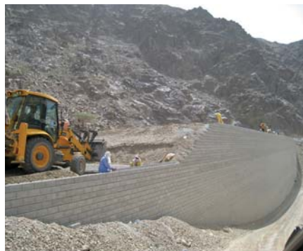
Facing units and geogrids are simple to install and as with all TensarTech Wall Systems connection to the face is easy yet secure.
