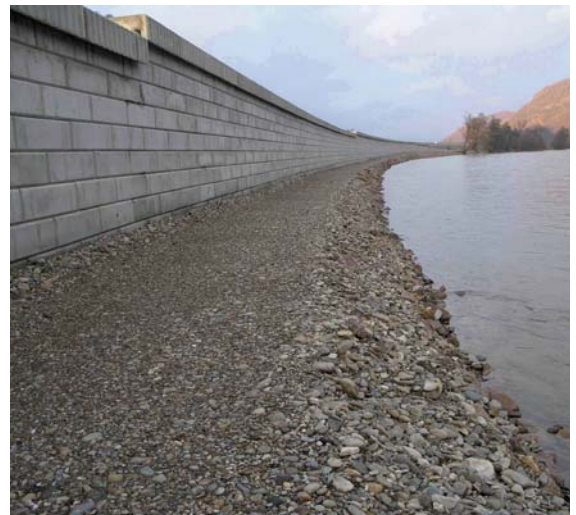
A TensarTech Marine System is well suited to aggressive coastal or tidal conditions such as harbour and river locations.
