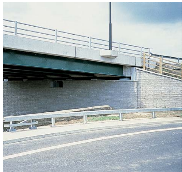
TensorTech Systems have been independently certified for use as load bearing bridge abutments in highway applications by the British Board of Agrément.
